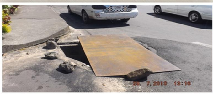
Figure 3: temporary slump cover in front of RSA
